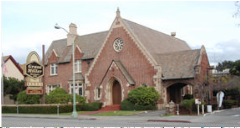
The same building in 2009. Four windows to the left of the entrance are the original residential windows.
