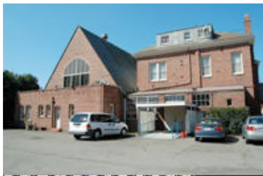
From the back, the shape of the original 1896 building is apparent on the right. Windows on the third floor testify that the third floor still exists; it is an apartment.
